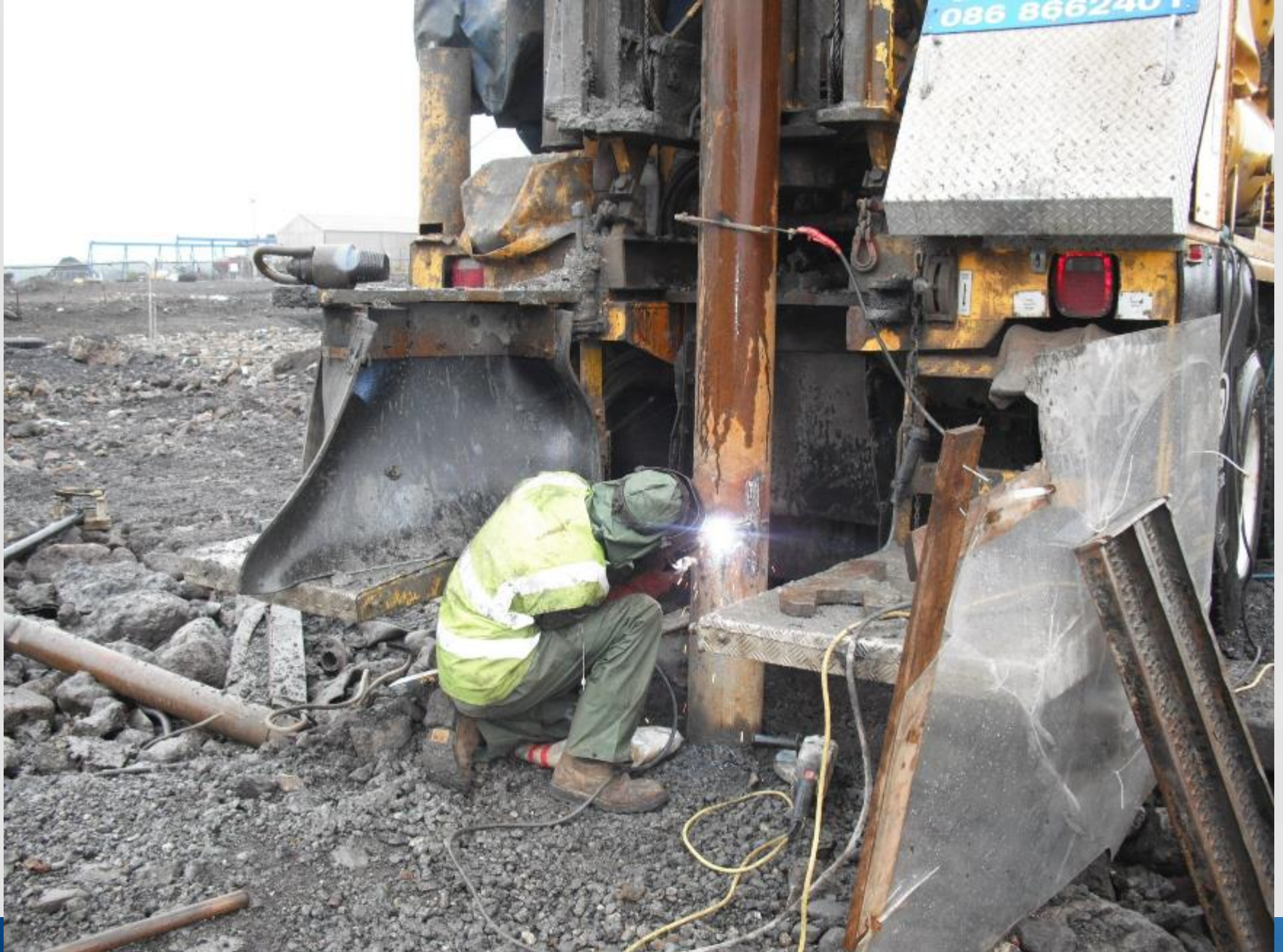
Haulbowline Island, Remediation Project
