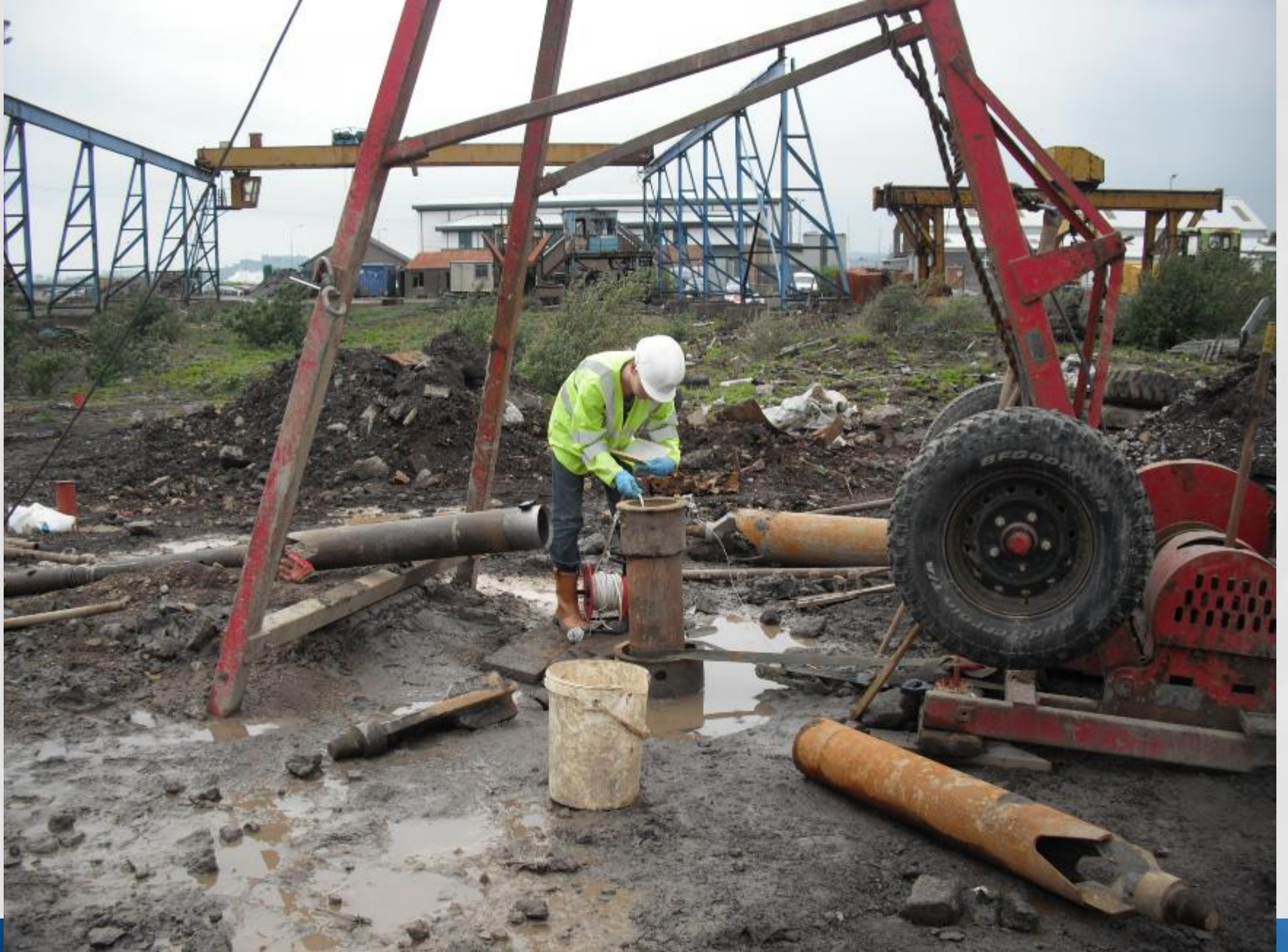
Haulbowline Island, Remediation Project
