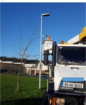
Installing the monitoring an existing lamppost
